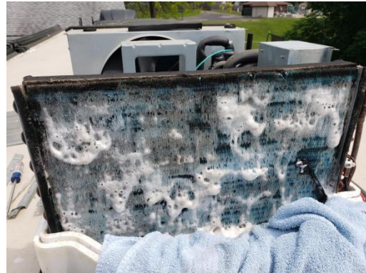
Picture of the evaporator with the "no rinse" cleaning foam applied
