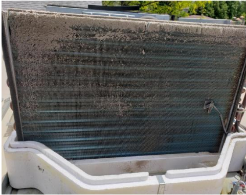
Picture of the dirty evaporator. This one is about two years since new. The other one was dirtier.
